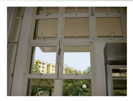
The SK-400 Electric operator in aluminum with linear rack movement, equipped with electronic limit switch, level of protection IP 30, posibility of connection in parallel, antidisturbance capacitor, complete with anodised aluminium bracket and window attachment in galvanised steel.
